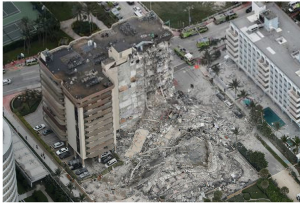
Part of the 12-story oceanfront Champlain Towers South Condo in Surfside, Florida, with more than 100 units, that collapsed on June 24, 2021. (Amy Beth Bennett/TNS)
