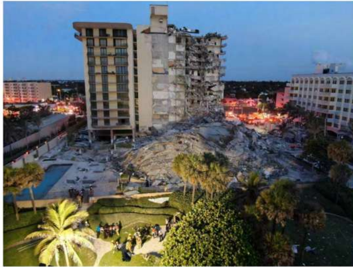
The partial collapse of the Champlain Towers South condo building that killed 98 people left a four-story tall pile of rubble. MIAMI
