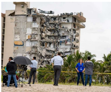
The collapse of Champlain Towers in Surfside killed 98 people and left dozens injured.
