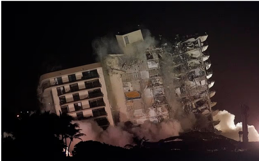
After the 2021 Surfside collapse (pictured), Florida cities have introduced stricter enforcement of building safety rules
